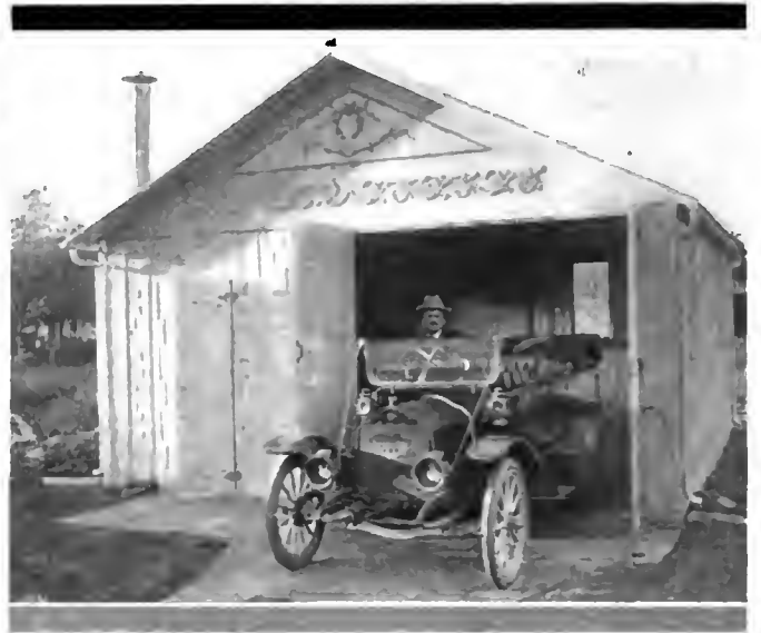
Fig. 4—Combined workshop and garage by the Metal Shelter Co. The equipment includes a forge with chimney, as shown
